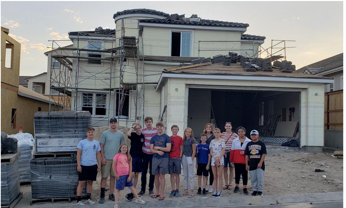
July 27 - YM/YW Career Night Home Construction
